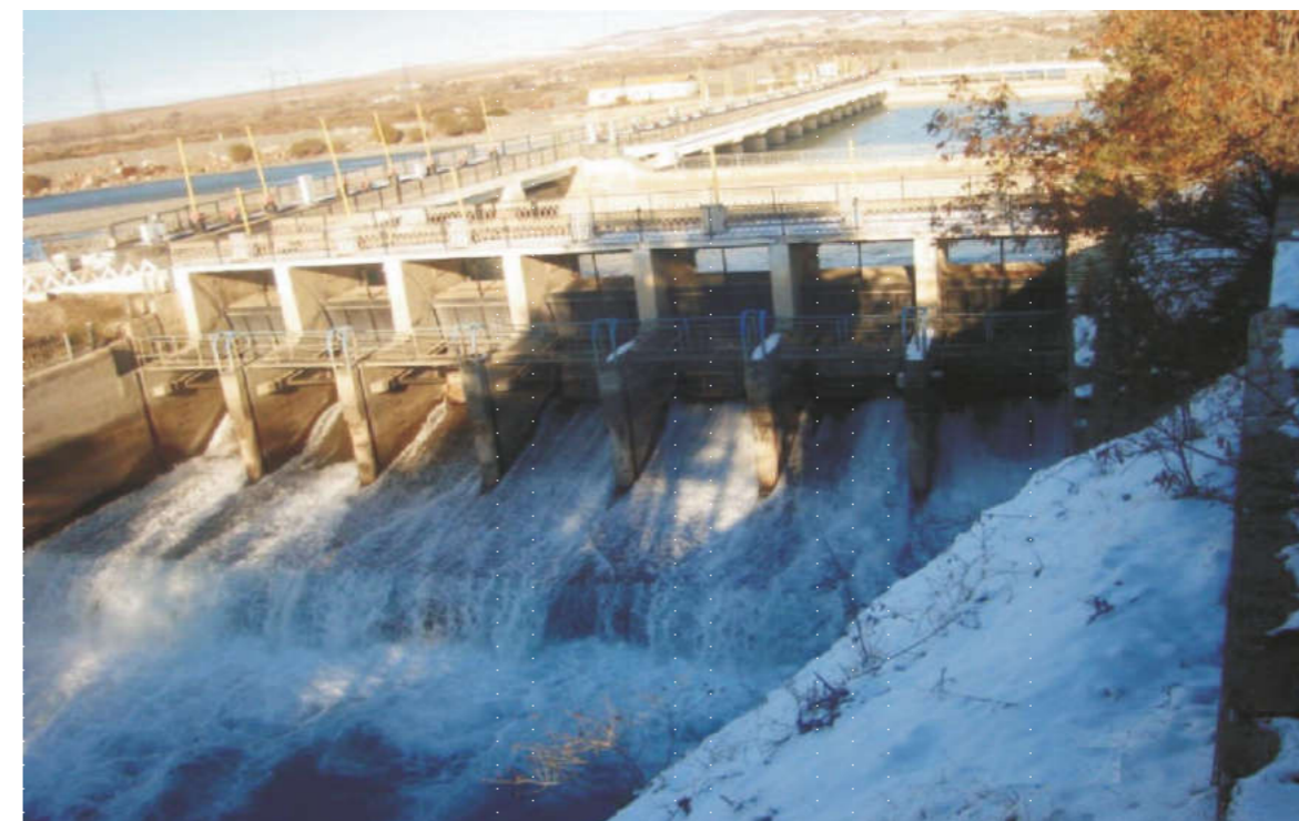
Figure 5. The Ravatkhodja Hydrostructure on the Zarafshan River
