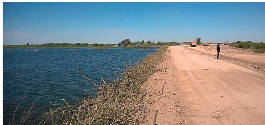
Fig. 2.9. Stopping Dam on the Maypost Lake (May 2017)
