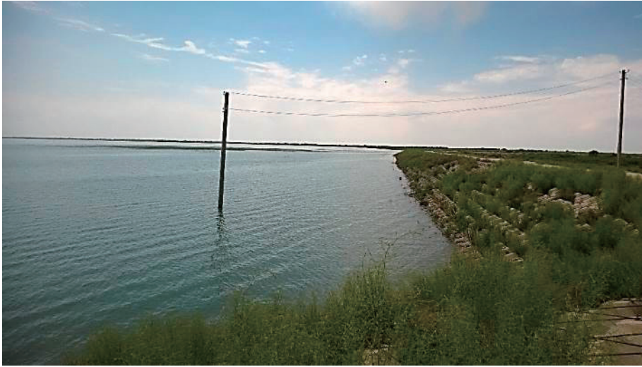
Fig. 2.6. Northern dam of Mejdurechensk reservoir, May 2017
