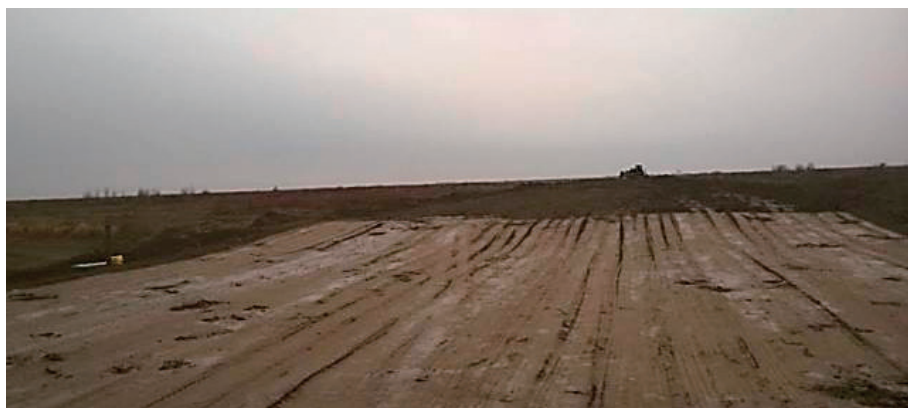
Fig. 2.7. Construction of the eastern dam of the Mejdurechensk reservoir; March 2017
